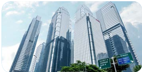
LANGHAM OFFICE 3 & HOTEL JAKARTA
