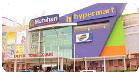
DEPOK TOWN SQUARE DEPOK
