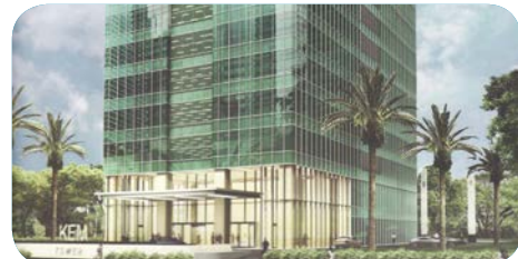
KEM TOWER JAKARTA
